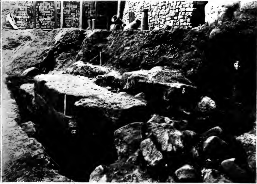
FIG. 3.—UPPER PORTION OF ROMAN WALL, LOOKING SOUTH. FOOTINGS NOT EXPOSED. a Ashlar work; b Rubble; d Footings of Wolf Tower.
